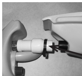
Photo 12 (Area where clamp is placed.)
